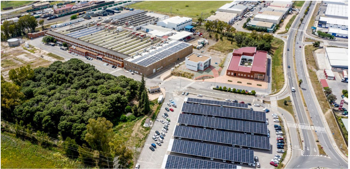
The Zafra site in Spain is the main component plant for the machining of DEUTZ engine parts. © DEUTZ
